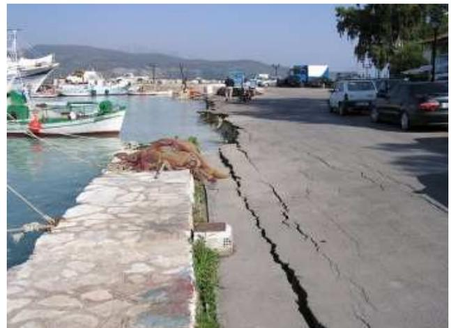
**Photos: Landslides and cracks in the port of Lygia after the earthquake of Lefkas (2003)**
